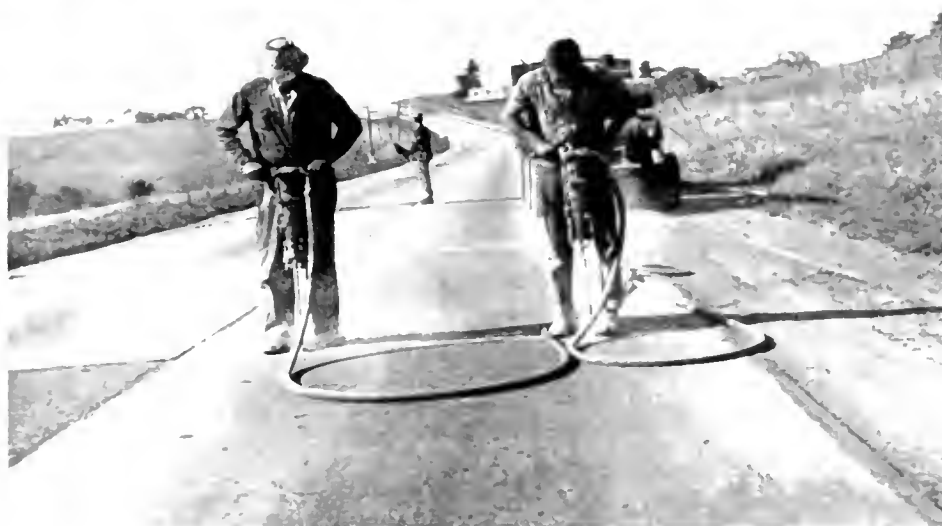
Upper—Mud jacking equipment in operation. Forcing cement treated loam under paving. Lower—Drilling holes preparatory to mud jacking operations
